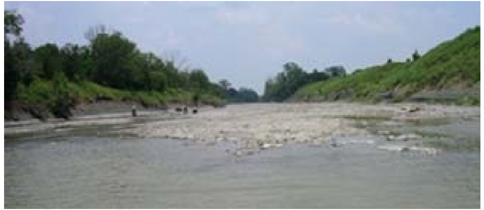
North Sulphur River at Highway 34
